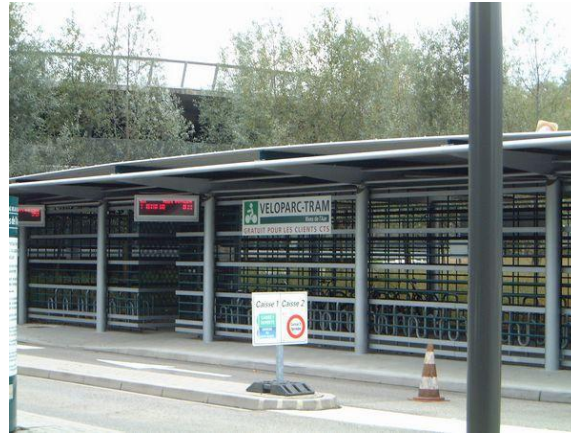
Covered bicycle parking tramway stops (Véloparc at Strasbourg)
