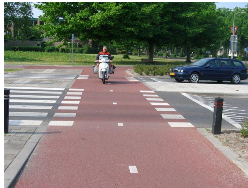
Two-way cycle lane crossing with traffic island with right of way (image source: P. Kroeze)
