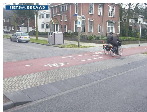
Cycle track crossing side road (image source: Fietsberaad)
