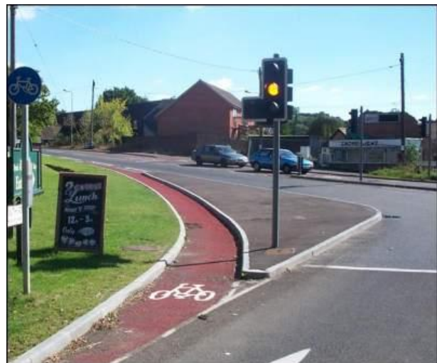
A cycling bypass past red – UK example (left-turn) (source: Cycling England, Rob Marshall)
