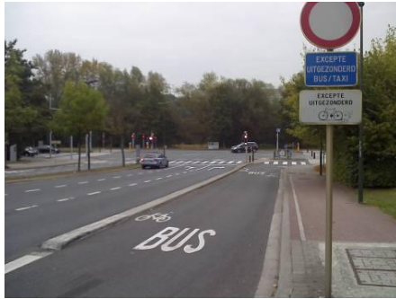
Bus/bike lane as a traffic light bypass for a right turn, with a closed profile and cycle road symbols (D. Dufour)
