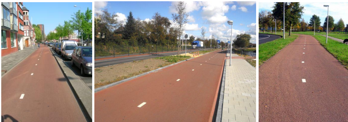
Two-way cycle tracks, on one side of a major road (image source: P. Kroeze)
