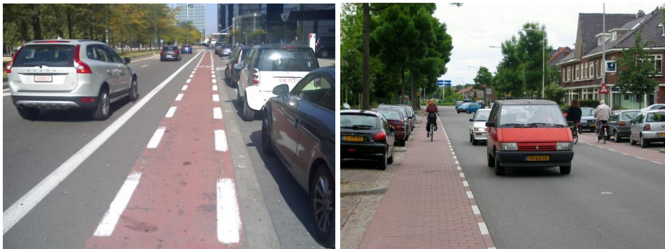
Cycle lane, at a safe distance from parked and driving cars (image source: D. Dufour)
